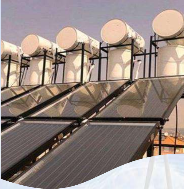
Roof Solar Heating Systems
